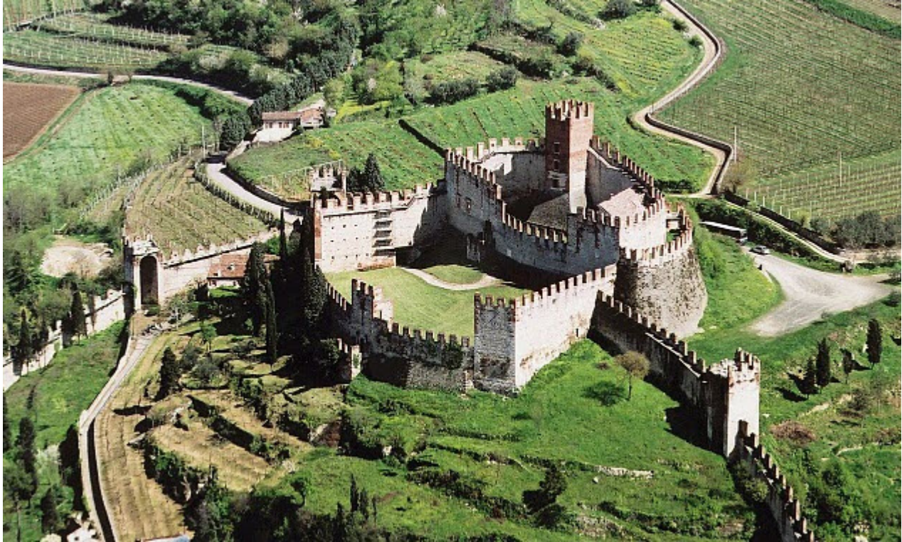
Aerial view of the Castello di Soave
